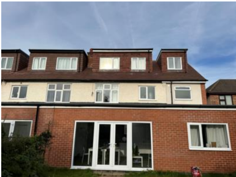
Rear elevation, no. 76 to the right
